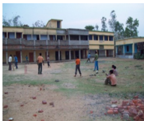
Polling Station Building Front View
