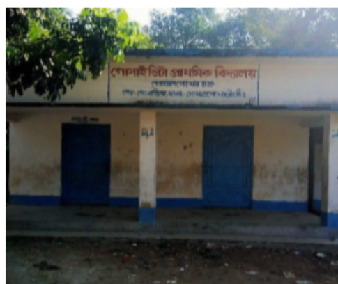
Polling Station Building Front View
