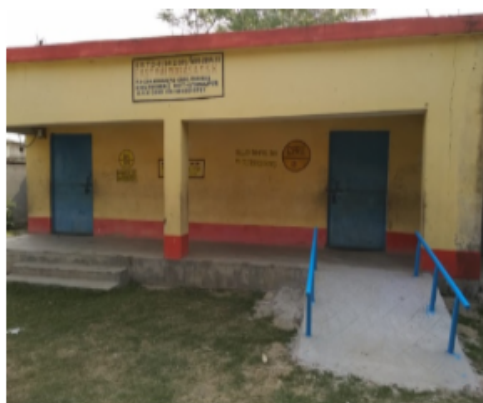
Polling Station Building Front View
