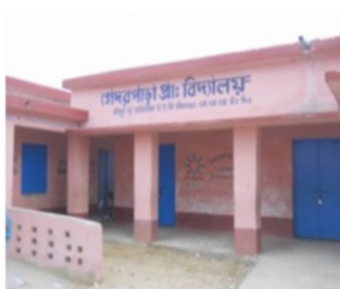
Polling Station Building Front View
