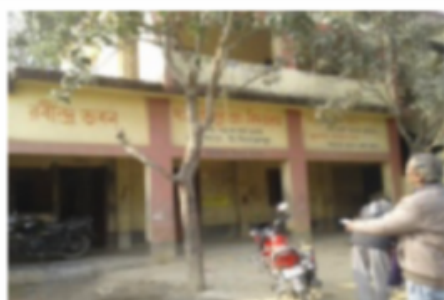
Polling Station Building Front View
