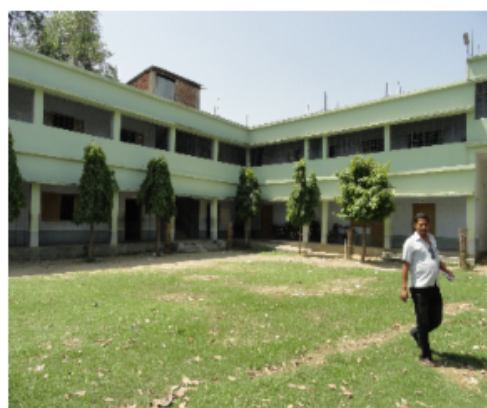
Polling Station Building Front View
