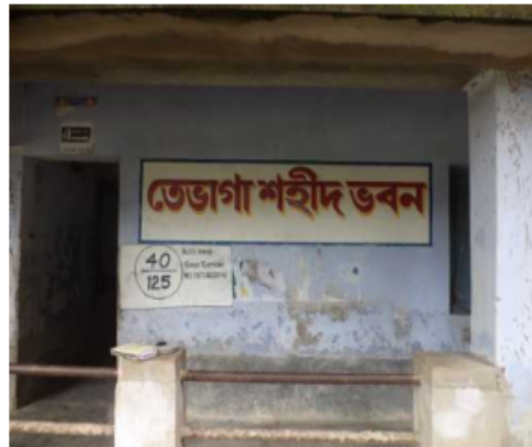
Polling Station Building Front View
