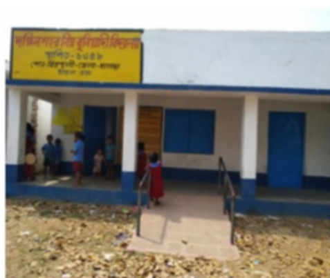
Polling Station Building Front View
