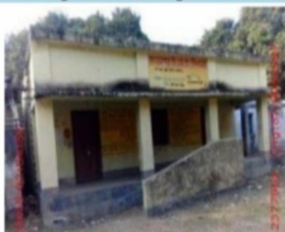
Polling Station Building Front View
