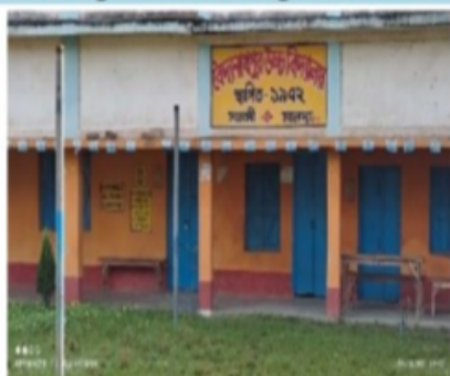
Polling Station Building Front View
