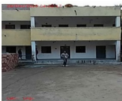
Polling Station Building Front View
