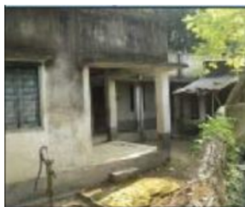
Polling Station Front View
