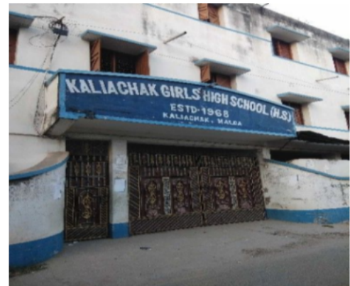
Polling Station Front View
