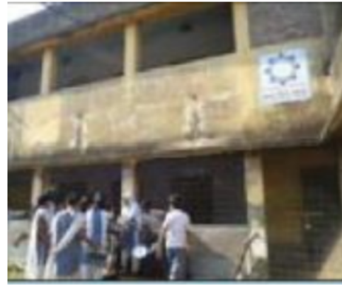
Polling Station Front View
