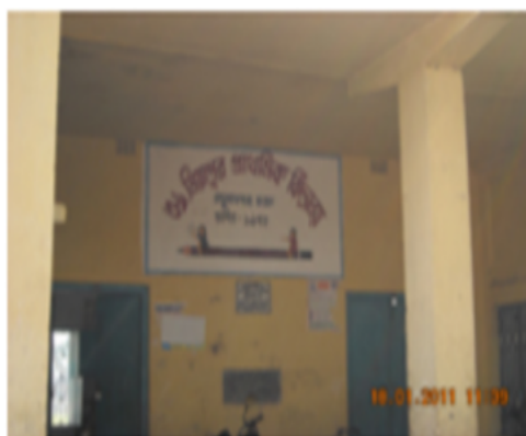
Polling Station Building Front View
