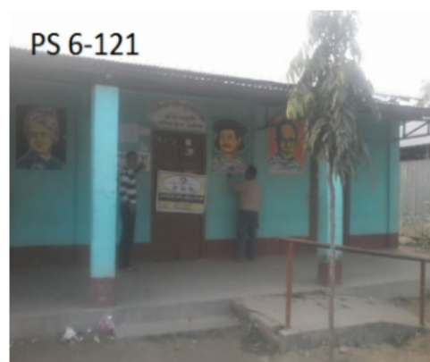
Polling Station Front View
