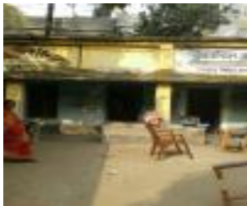
Polling Station Building Front View
