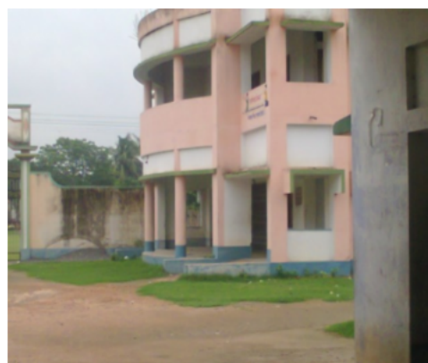
Polling Station Front View
