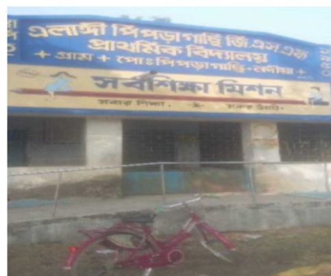
Polling Station Front View
