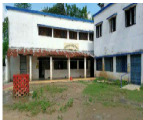
Polling Station Front View
