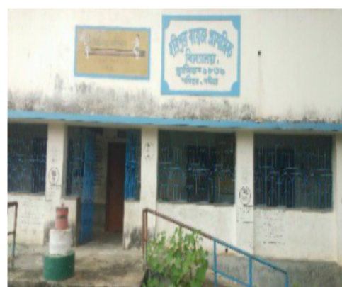
Polling Station Front View
