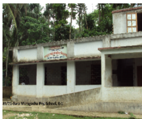
Polling Station Building Front View
