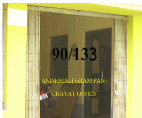
Polling Station Building Front View
