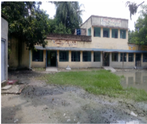
Polling Station Building Front View
