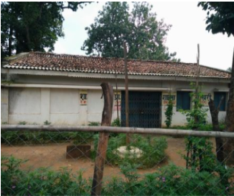
Polling Station Building Front View
