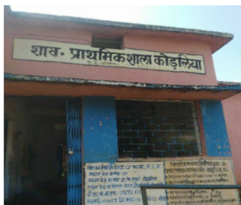
Polling Station Front View
