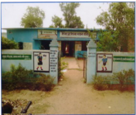
Polling Station Front View
