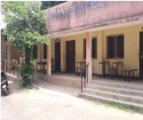
Polling Station Front View
