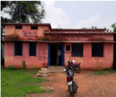
Polling Station Front View
