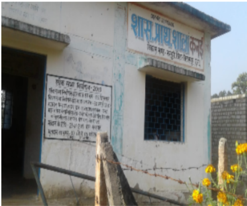
Polling Station Front View
