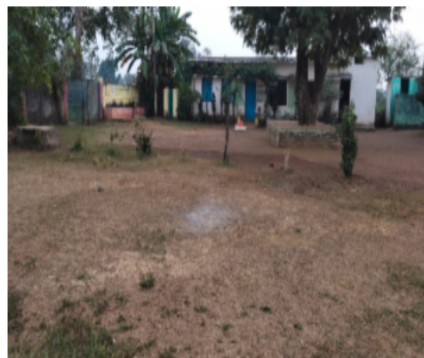
Polling Station Front View
