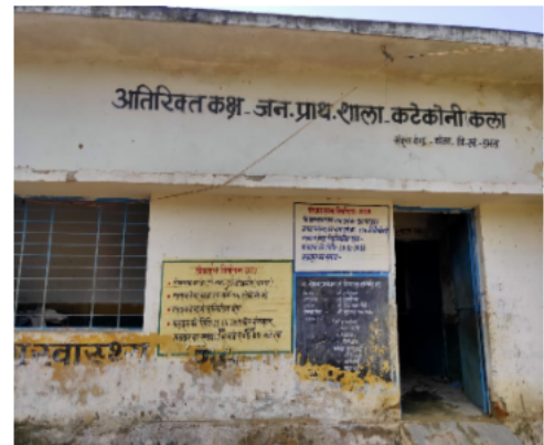
Polling Station Front View
