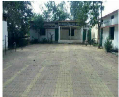
Polling Station Front View
