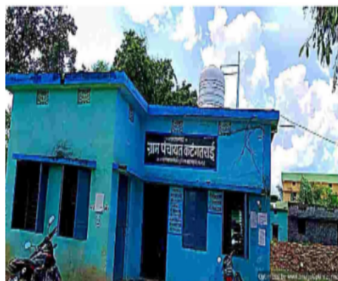
Polling Station Front View
