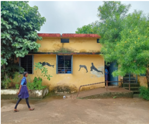
Polling Station Front View
