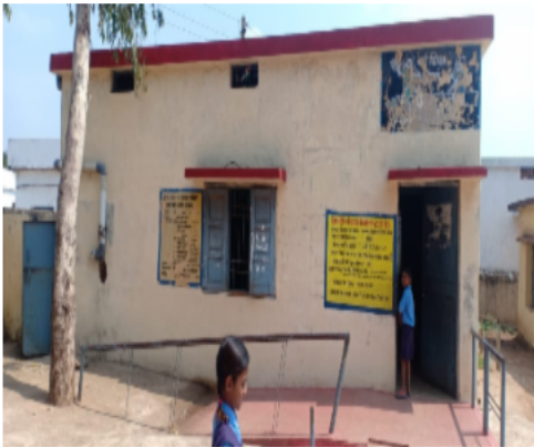
Polling Station Front View
