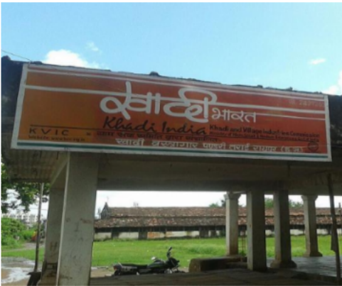
Polling Station Building Front View
