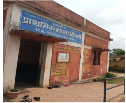
Polling Station Front View
