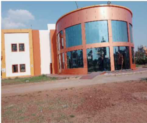
Polling Station Building Front View
