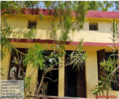
Polling Station Building Front View
