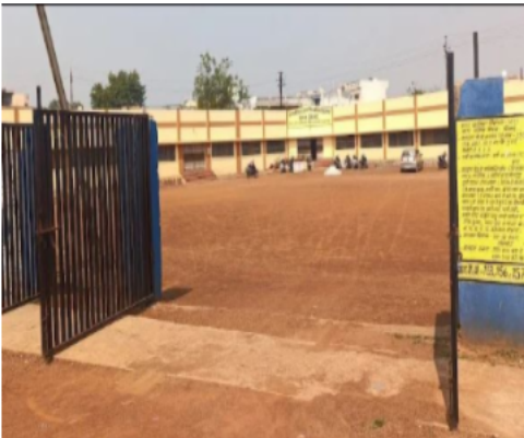
Polling Station Building Front View
