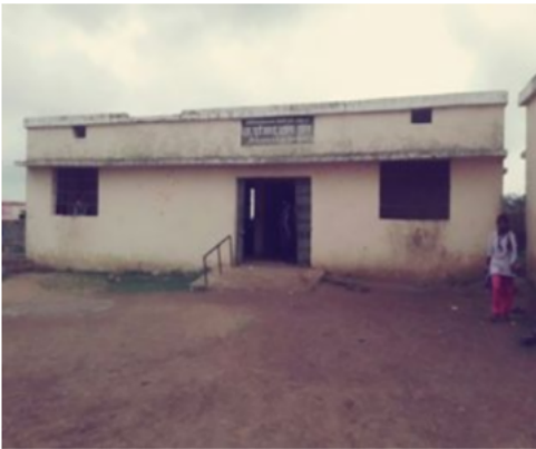
Polling Station Building Front View
