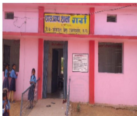
Polling Station Front View
