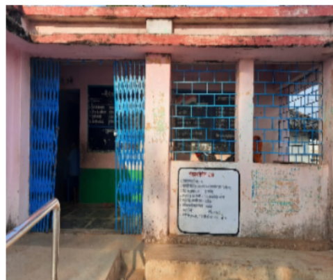
Polling Station Front View
