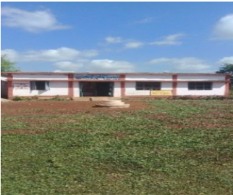
Polling Station Building Front View
