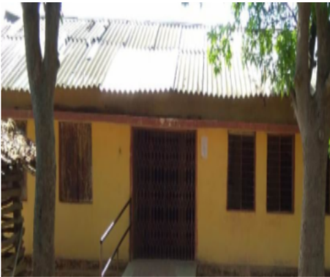
Polling Station Building Front View
