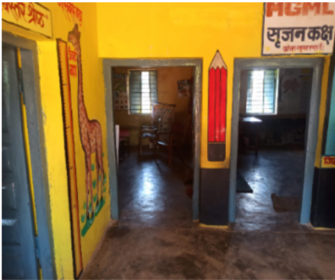
Polling Station Front View
