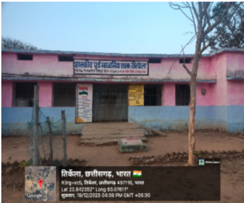
Polling Station Front View
