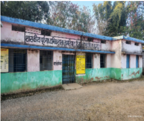
Polling Station Building Front View
