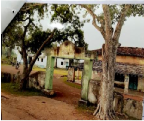
Polling Station Building Front View
